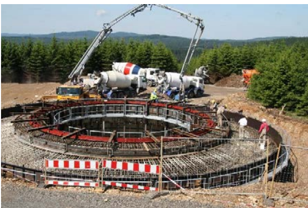
Picture 3 Foundation of windmill
