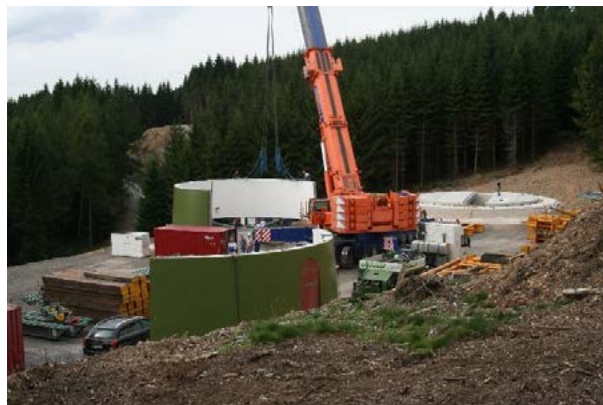
Picture 4 Construction of windmill
